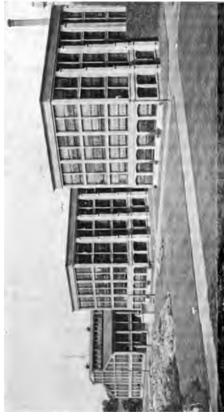
Fig. 3. United Shoe Machinery Plant, Beverly, Mass. These buildings may be taken as models of factory construction. They are of fire-resisting material, moderate height, and have liberal light-courts, with a window area of approximately 30% of the floor area.
